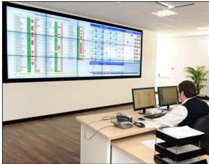
The newly refurbished WSC control Centre – 2012
